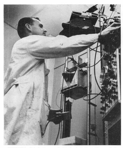
OUTCOME of test of a sample block of urethane foam will be recorded on oscilloscope and observed by Ernest R. Dunaway.
